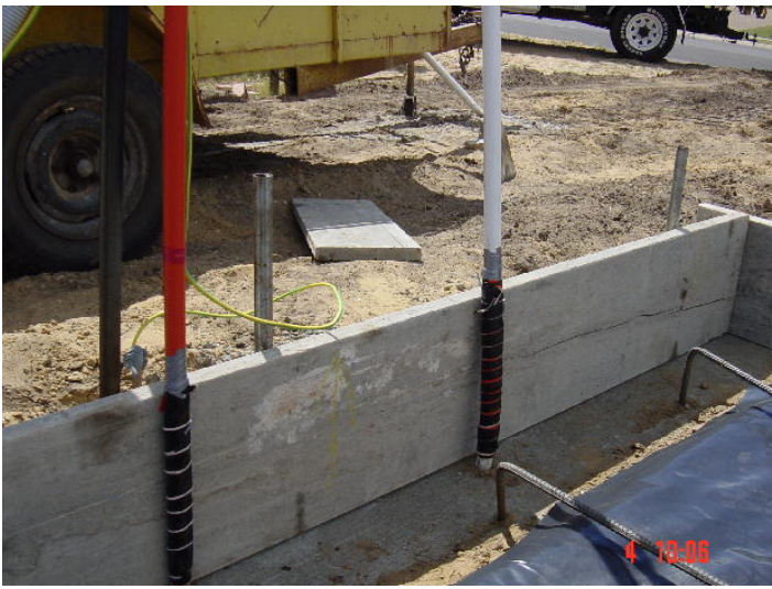
photo 1 before the slab pour showing black plastic facing out large overlaps
